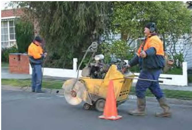
Figure 20: A concrete saw. Concrete saws frequently used in road maintenance activities can be a large source of stormwater pollution if precautions are not taken. (Paris, Josh. 2007.)
