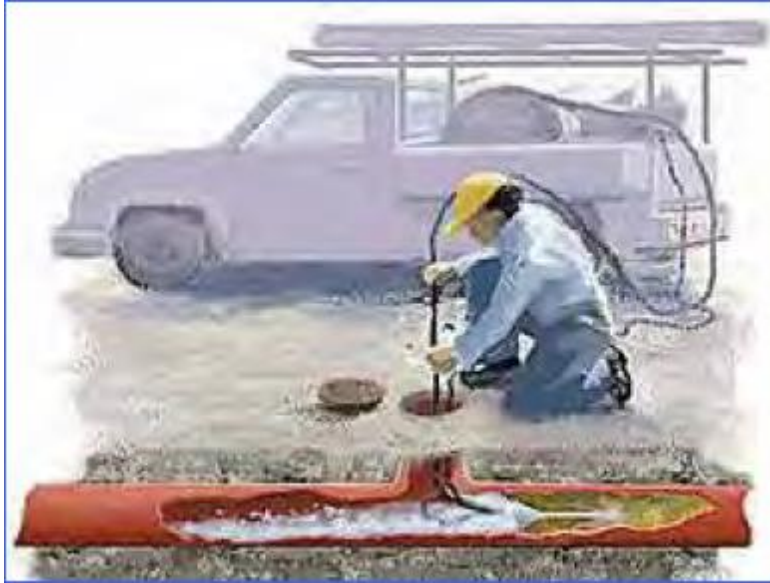
Figure 29: Storm pipe cleaning using the flushing method. Storm drains and pipes should be cleaned at least once a year to remove debris that has collected in the drain. (Office of Water. 2009.)
