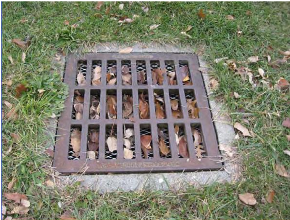
Figure 31: Catch basin with smaller grate size to catch leaves. Catch basins have varying grate sizes. Some jurisdictions use grates with smaller holes or catch basin inserts to trap smaller debris. The drawback is they require cleaning more often for efficiency. (See reference 27.)
