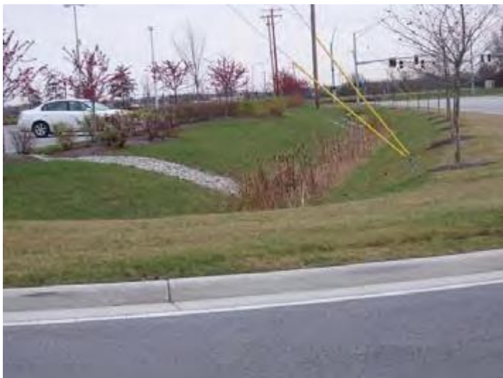
Figure 23: Example of a Bioswale. (English, Jennifer. 2009. Defiance Soil and Water Conservation District)
