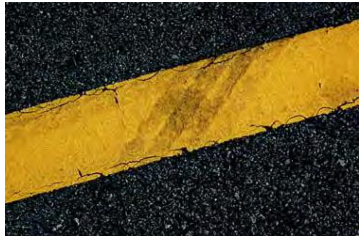
Figure 21: A yellow road stripe. Road striping is necessary for driving, but to protect stormwater, striping should only be performed on clear days with little wind. (Tan, Sherman. 2007.)
